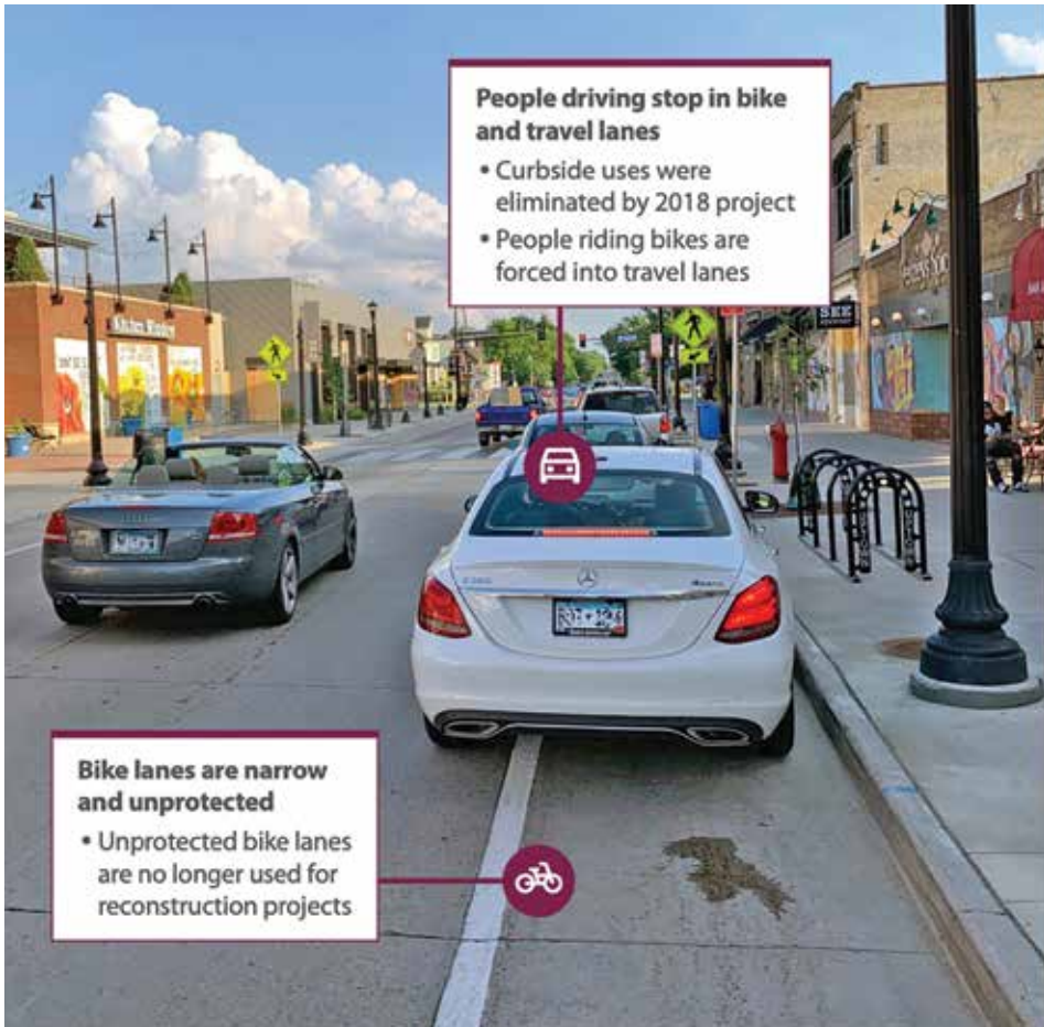
Existing design challenges on Hennepin Avenue (Image: City of Minneapolis)
